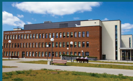
LSMU Emergency centre
